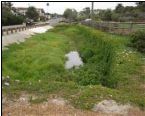
Figure 2. Cottonwood Creek (Upstream)
