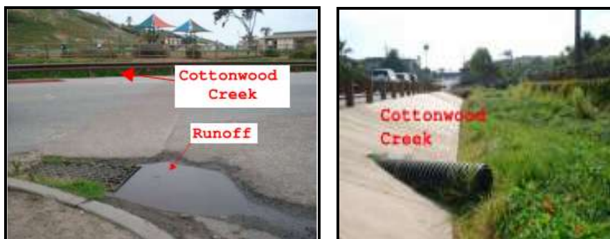
Figures 9 & 10 Residential Runoff into Cottonwood Creek
