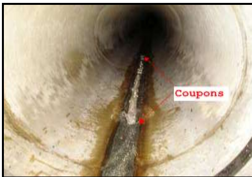
Figure 5. CSD037 (upstream, below manhole)
